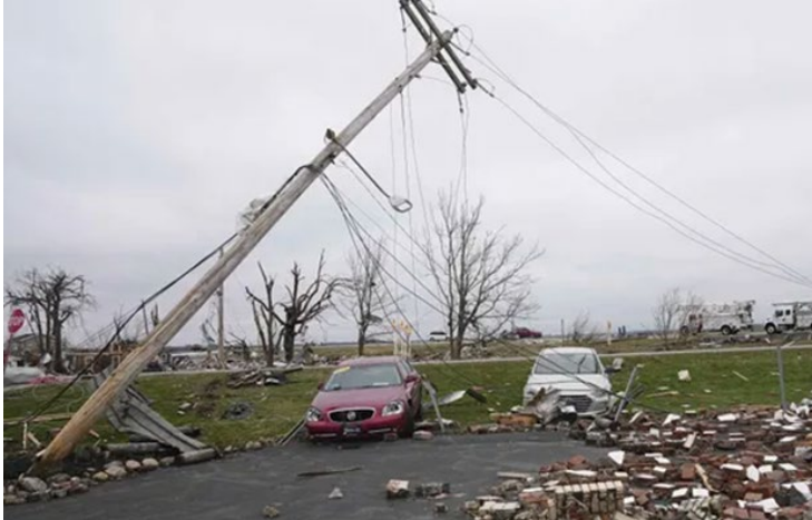
Figure 4: Downed power line
